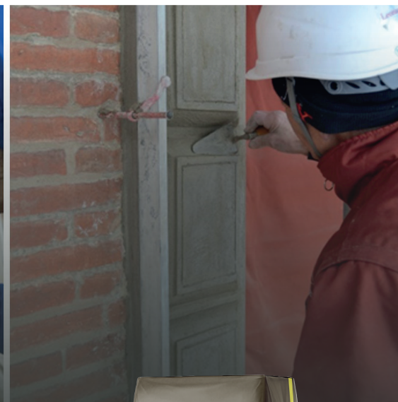
APPLICATION SHEET Stone repair
